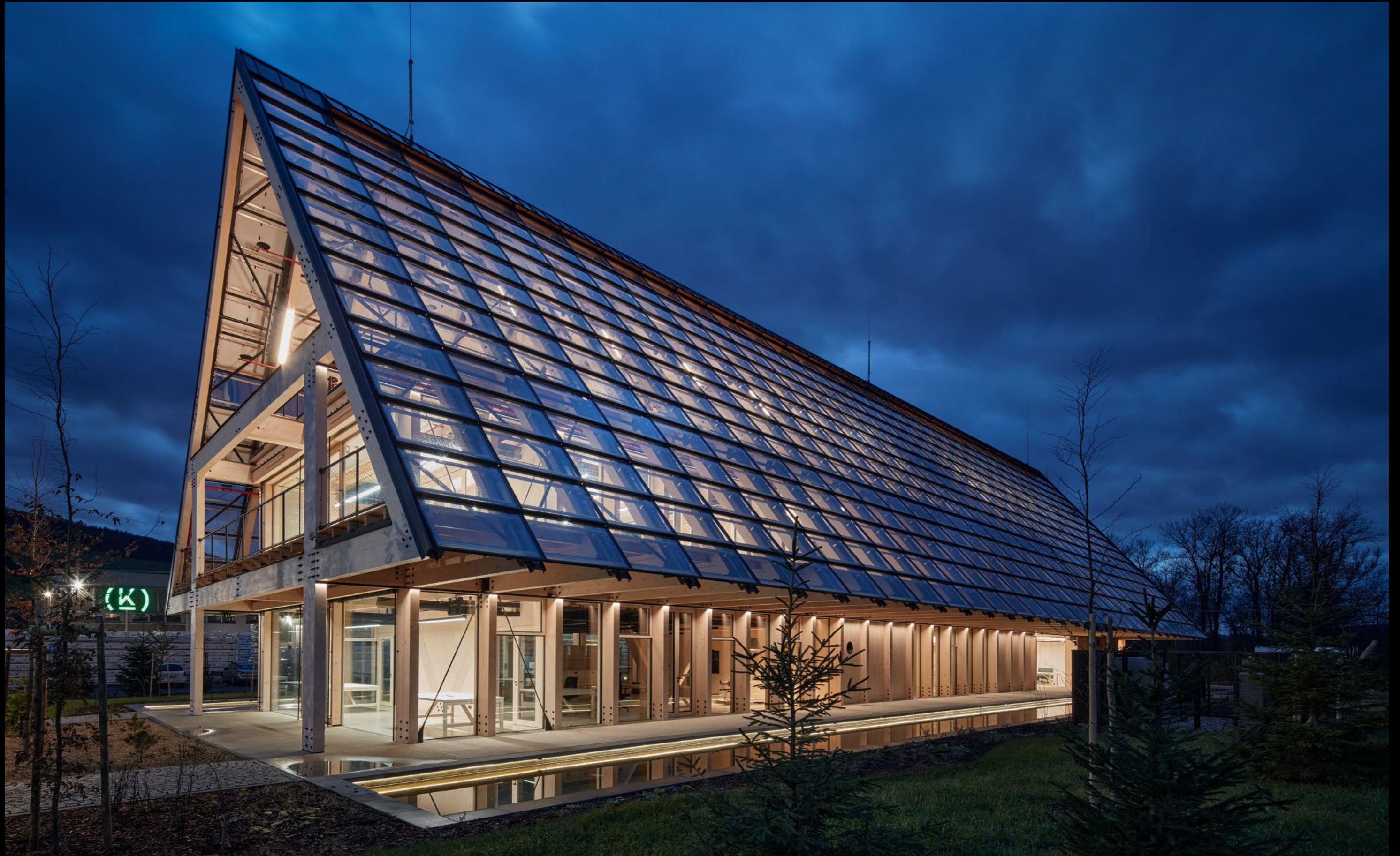
A clever and clear design: While on the north side of the building the wooden structure is exclusively covered with glass panels, more than half of the south side is covered with photovoltaic modules (photo: BoysPlayNice)
